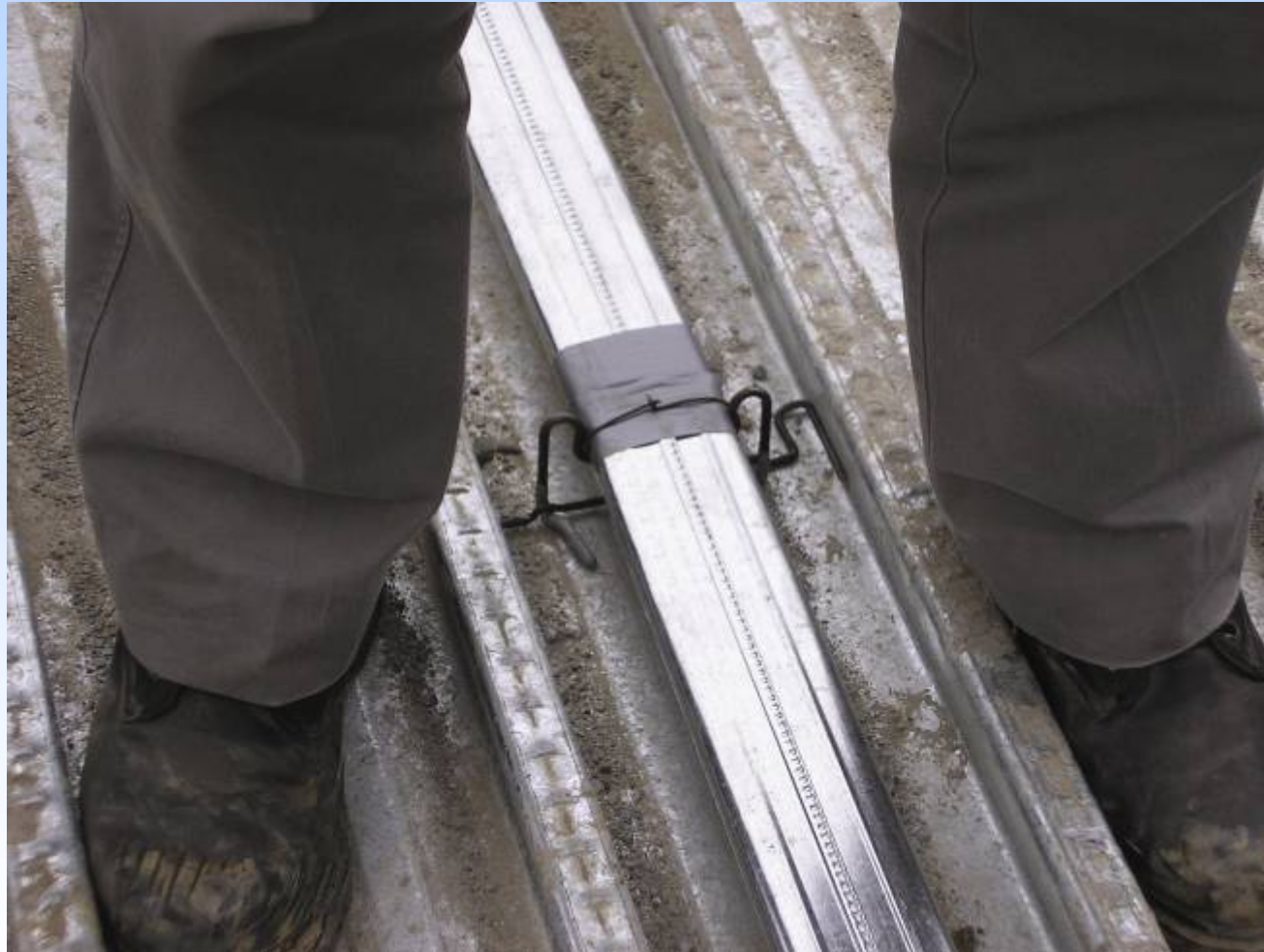
P-T tendon between ribs
