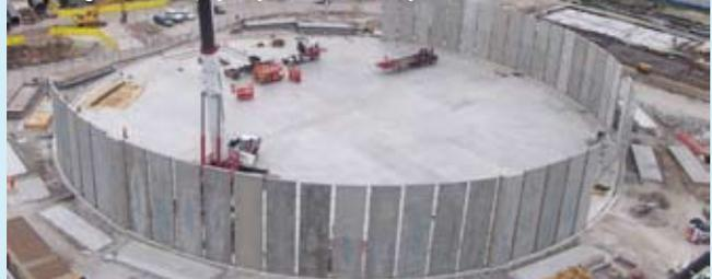
PT slab for its foundations to accommodate the high static and rolling loads. The use of a 350 mm thick PT slab is in contrast to the 1000 mm thick slab (at footings) in an earlier pilot plant.
