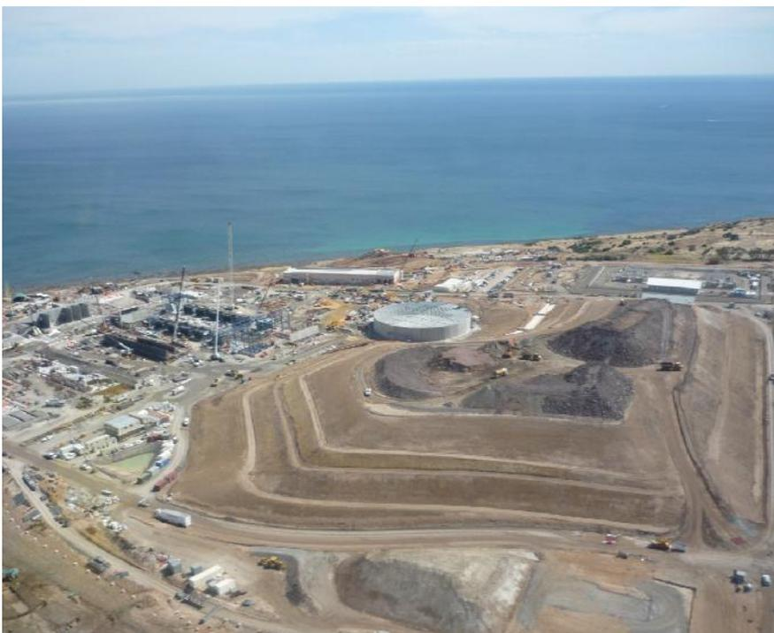
An important part of the Adelaide Desalination Project is the transfer pipeline system to deliver water from Port Stanvac to the Happy Valley water treatment plant with these Treated Water Reservoirs feeding this system. Desalinated water will be pumped through the pipeline to Happy Valley where it will be combined with water from the water treatment plant before entering the existing water supply network.
