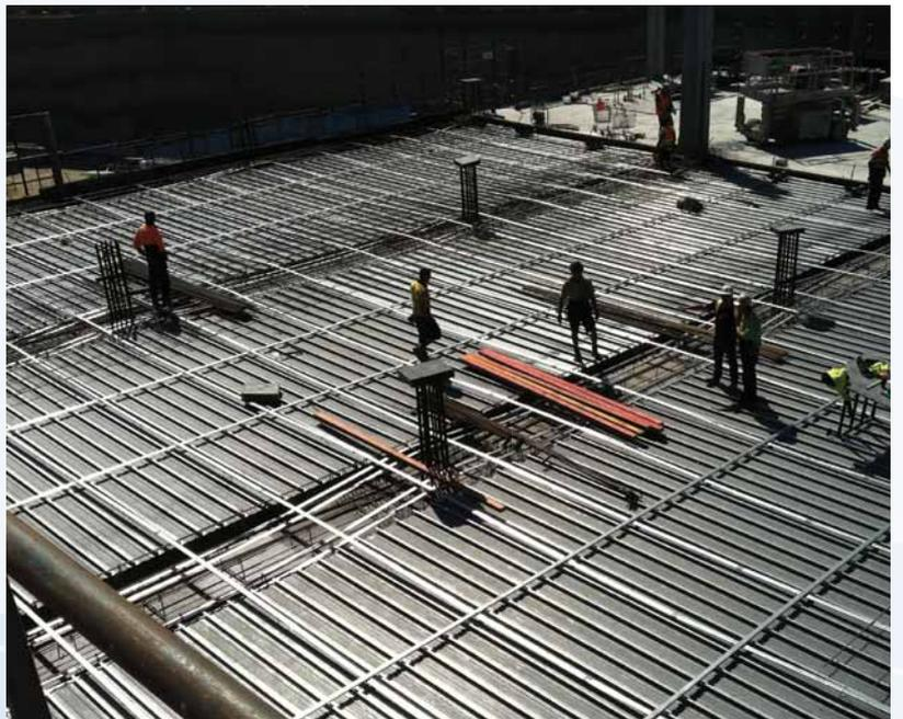
As the post-tensioning contractor on the project, AusPT's involvement consisted of three levels of suspended post-tensioned floors for various retail and car park occupancy.
