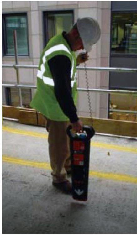
**Fig 4 – Locating and marking tendons on the top surface.**
